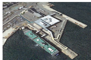
Ryotsu Port (Minato District) Quay (-7.5 m) (Seismic-Resistant)
