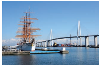
Fushiki-Toyama Port Shinminato Bridge
