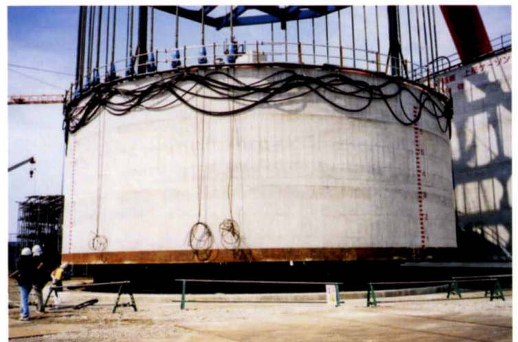
Appearance of the suction foundation (RC)
